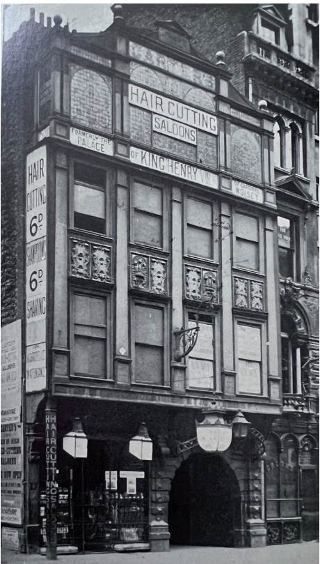
No.17 Fleet Street before restoration
